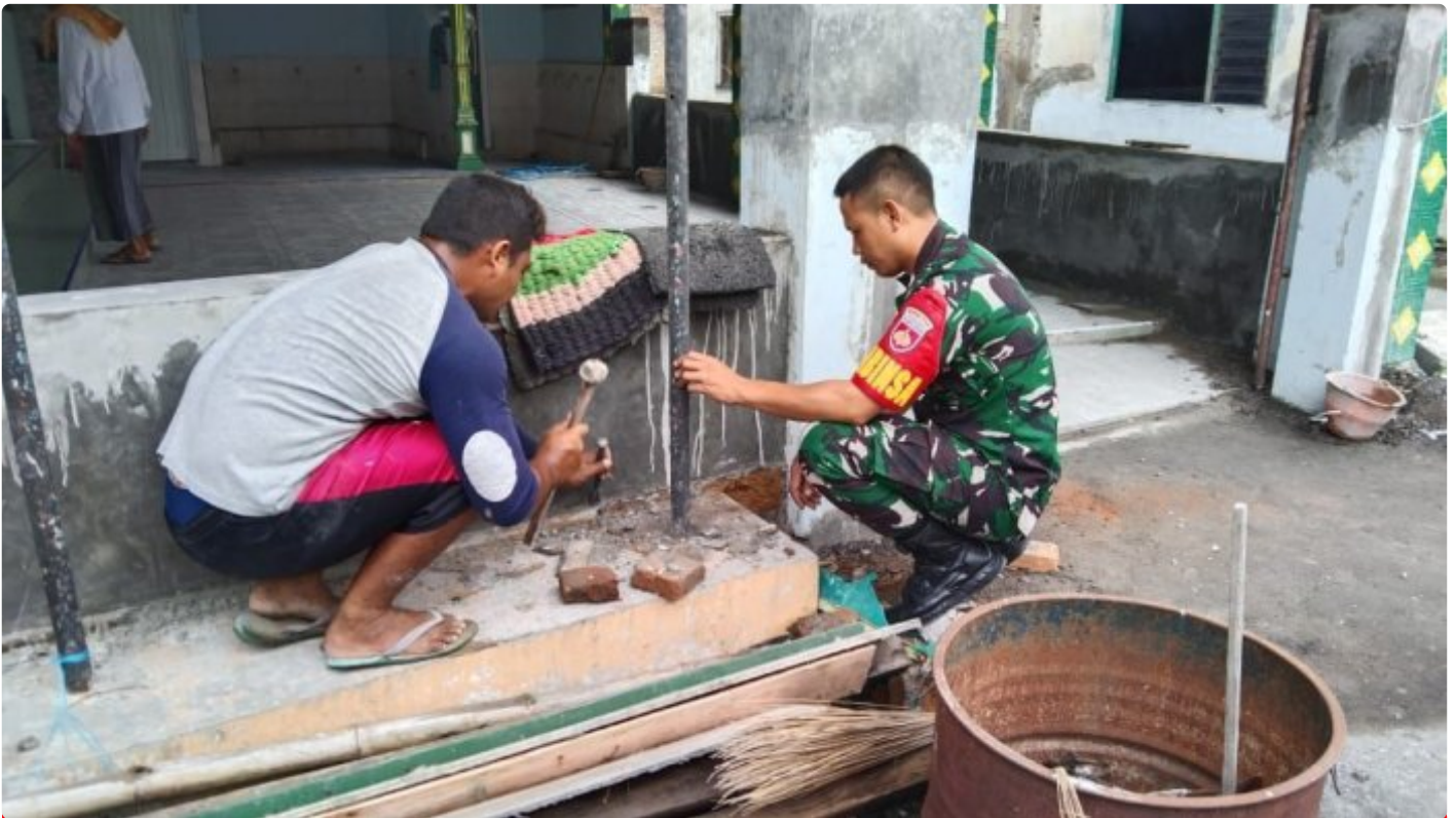
Babinsa Ceper Monitoring Rehab Masjid Di Dukuh Pason
